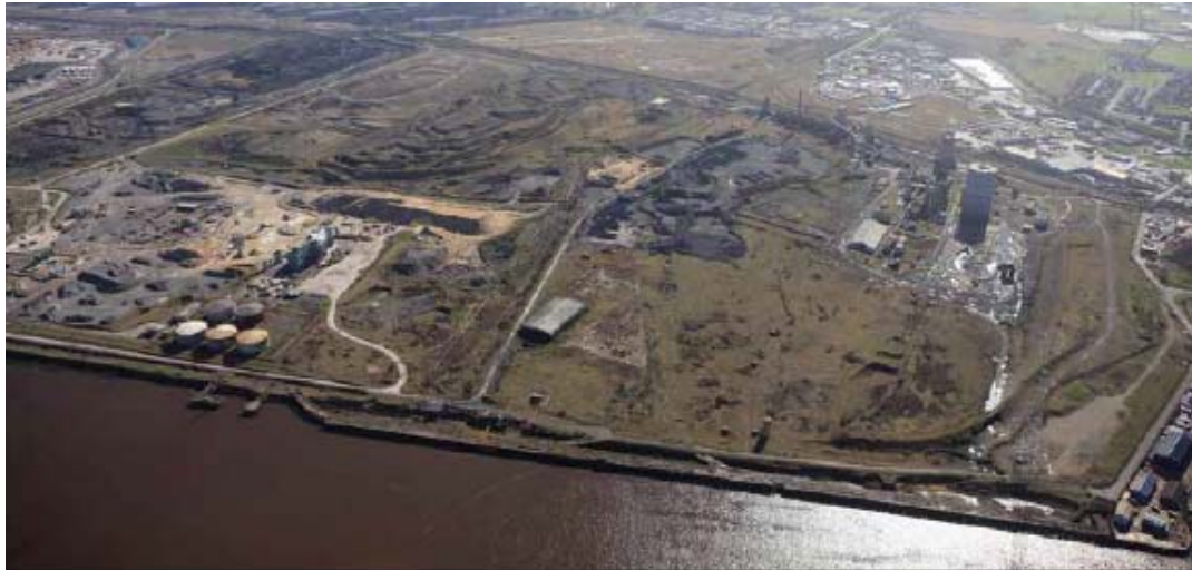
Figure 2.1 Aerial view of application site
